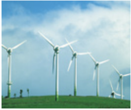
■ ALTERNATIVE ENERGY SUPPLY TECHNOLOGIES
